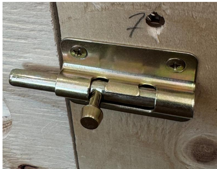
Figure: Barrel Bolt Installation
